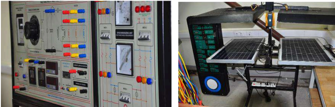
Power Systems Lab, Left: Alternator Fault Simulator wWith Grid Synchronization Facility, Right: Solar Photo Voltaic Array Simulator
